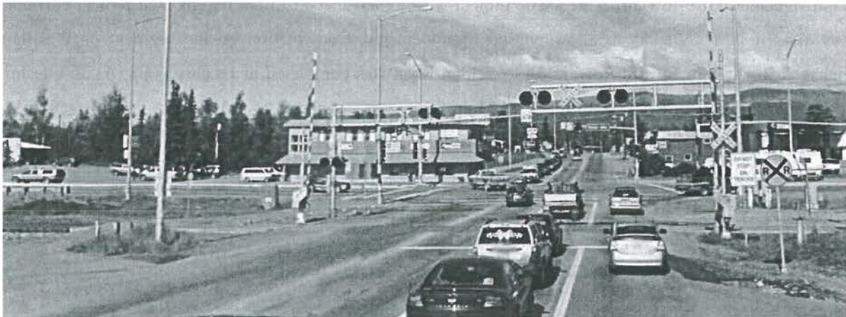
KGB Road @ ARRC crossing – facing north towards Parks Highway
